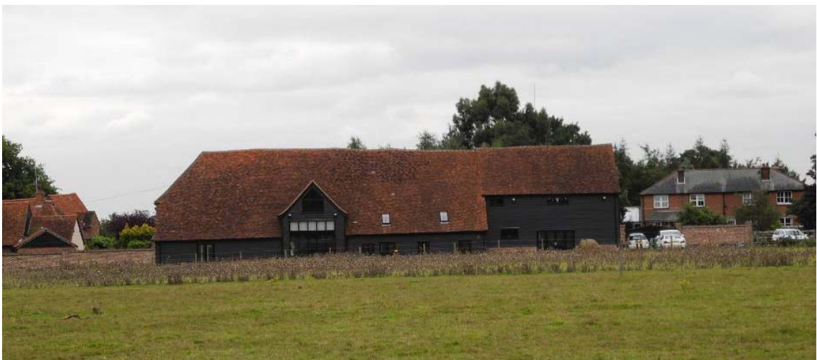
Fig. 17 Fryerning Hall Barn from Beggars Hill. Fryerning Hall Cottages are to the right of it
