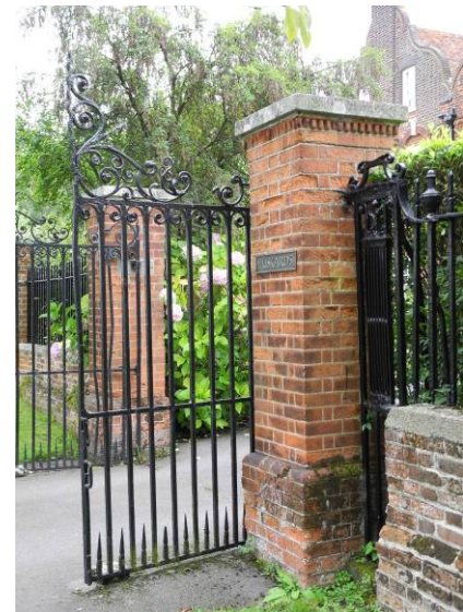
Fig. 8: Wrought iron gates at Huskards
