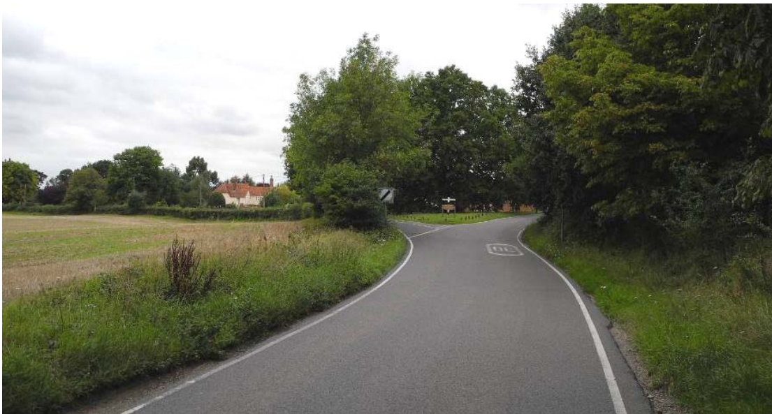
Fig. 10: Junction of Fryerning Lane and Blackmore and Mill Green Roads at Church Green, with view to Fryerning Hall
