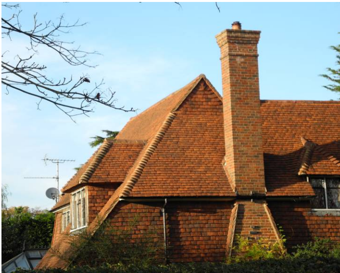
Fig. 7: Typical features of Arts and Crafts styling, big cat-slide roofs, dormer windows, tile hanging, chimneys, and metal windows with leaded lights, seen here at Draycott House, Back Lane
