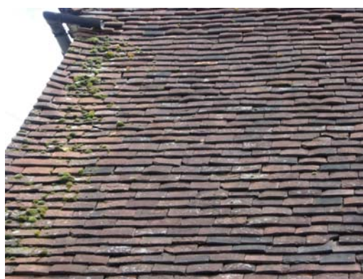
Fig. 9 Plain clay roof tiles.
