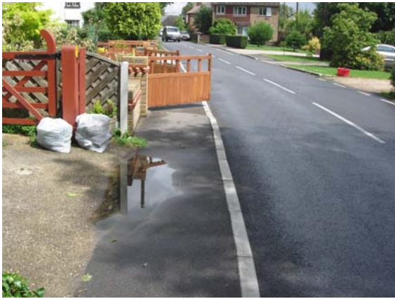
Fig. 12 Tarmac with concrete kerb stones, Blackmore Road.
