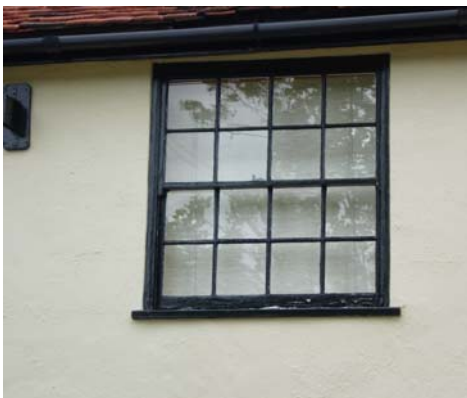
Fig. 8 Original timber window.
