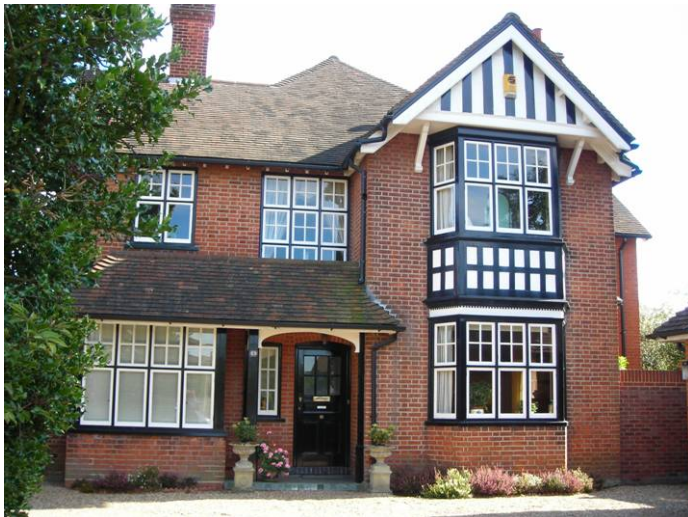
Figs 18 & 19 No. 69A High Street (above) and no. 69 High Street (left).
