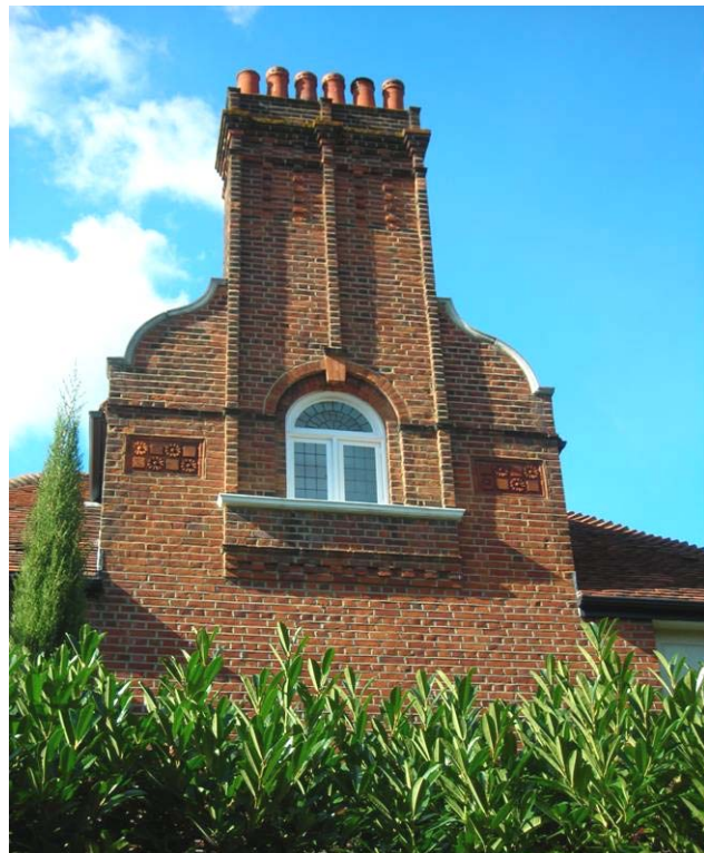
Fig. 16 English bond brickwork, The Gate House.
