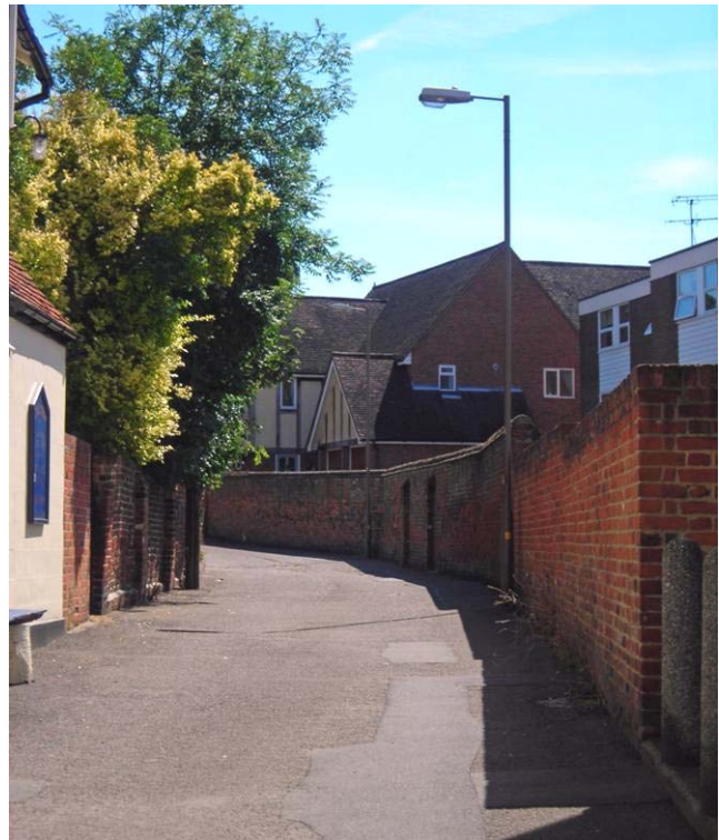
Fig. 30 Red brick boundary walls, Star Lane.
