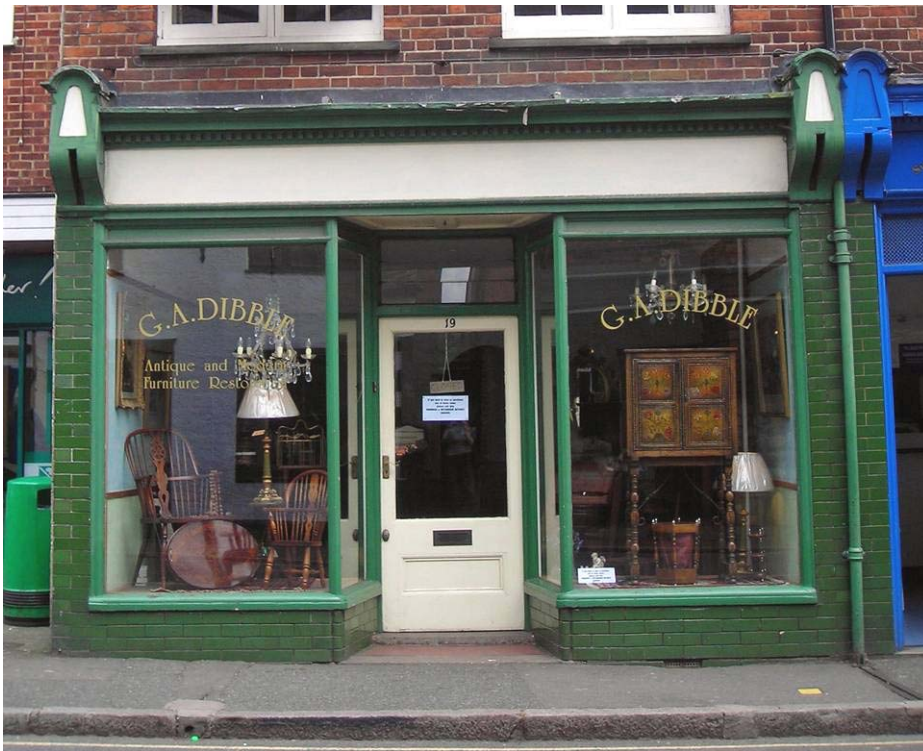
Fig. 29 Traditional shop front with green glazed brick surround, central recessed door and moulded consoles, no. 19 High Street.
