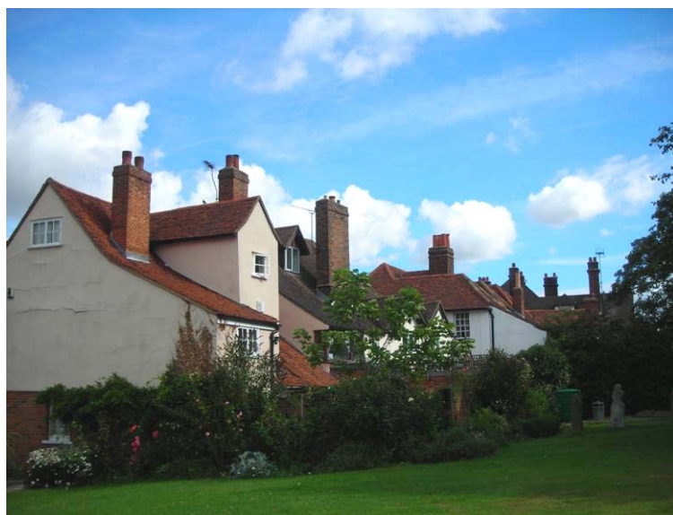
Fig. 26 Clay roof tiles and brick chimney stacks contribute to a lively roofscape in this view from the churchyard.
