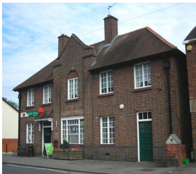
Fig. 77 The Post Office. A portion of the boundary wall of the old Victorian infant school survives to the right.
