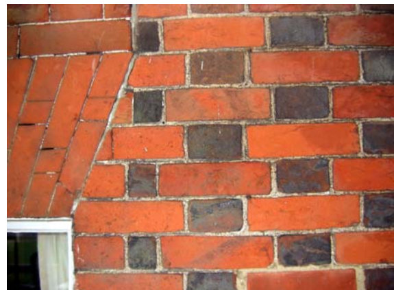
Fig. 14 Georgian brickwork with flared headers and penny-struck pointing (Roden House, Shenfield Road).
