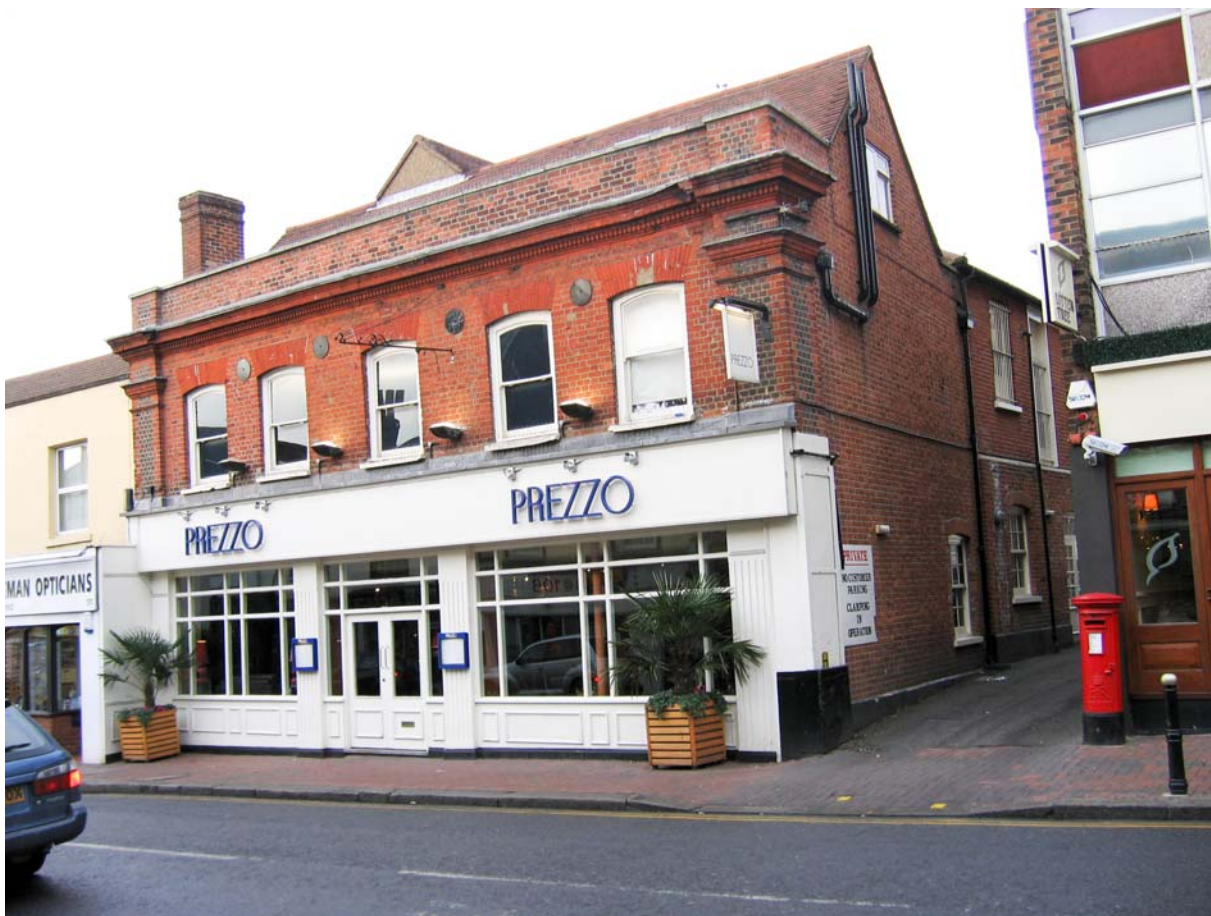
Fig. 41 Nos 129-129a High Street, late 18th-century brickwork with classical detailing encasing an older timber frame.
