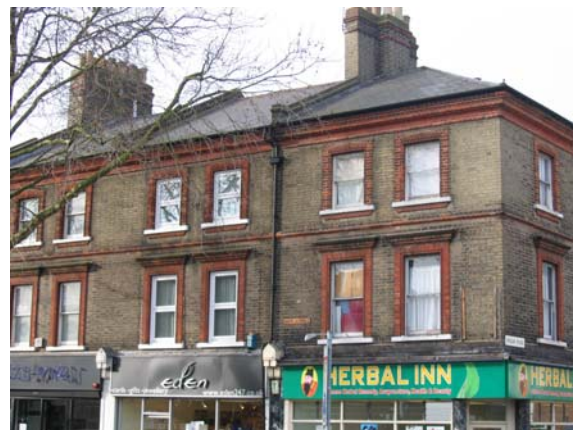
Fig. 15 Yellow stock brickwork with red brick detailing at nos 1-23 High Street.
