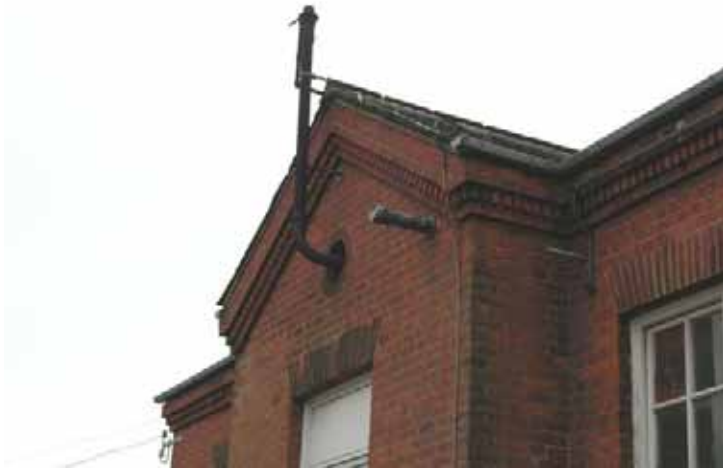
Fig. 12 Flemish bond brickwork showing brick arches and denticulated eaves
