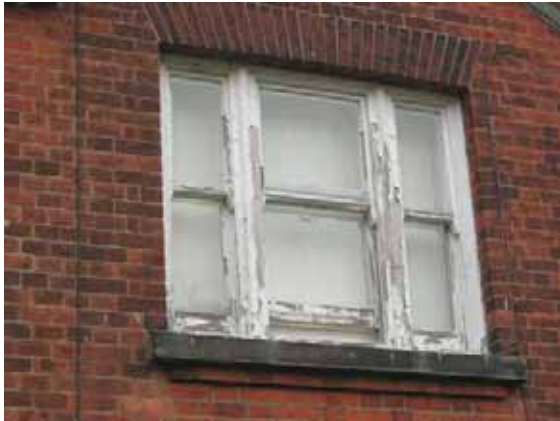
Fig. 59 general condition of windows throughout the site
