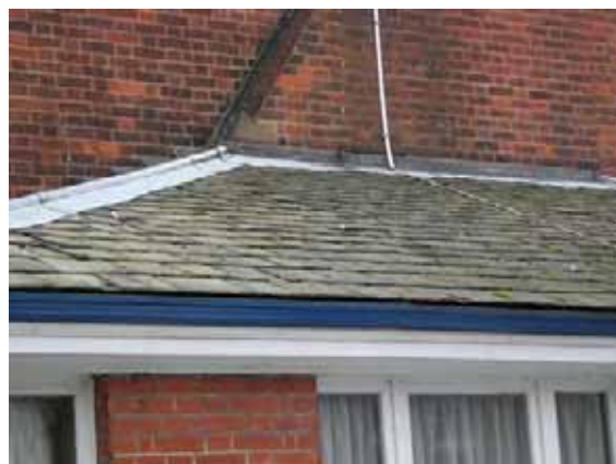
Fig. 7 Example of slate roof
