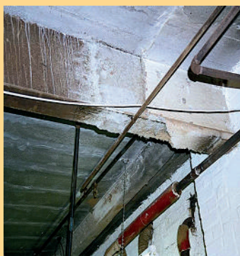
Sprayed Asbestos and Lagging.
