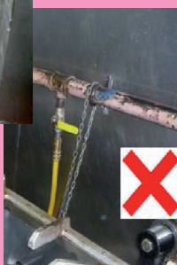
Restraining wire attached to the pipework
