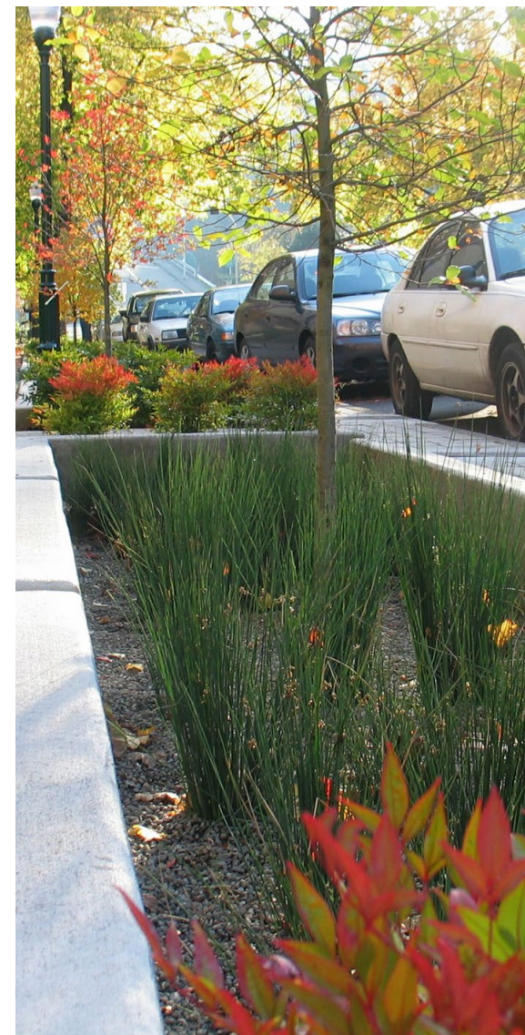
Bio-retention planters, Portland, Oregon, USA
