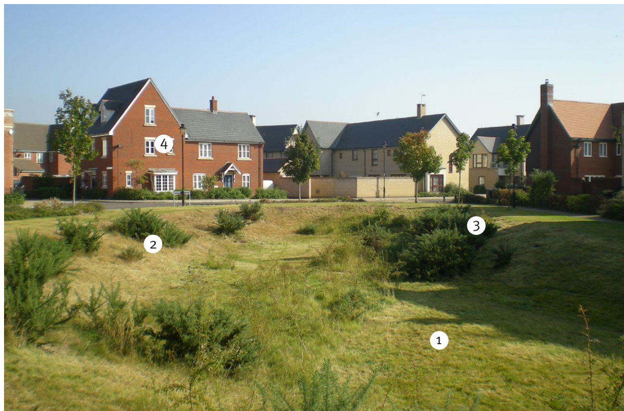
Infiltration basin at Ravenswood
