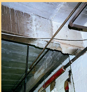
Sprayed Asbestos and Lagging.
