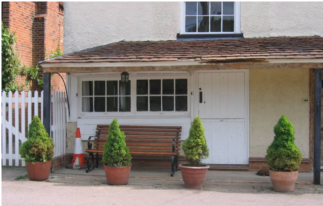
Fig. 12: Former butcher's shop window with top- and bottom-hung shutters (21 Cricketers Lane).
