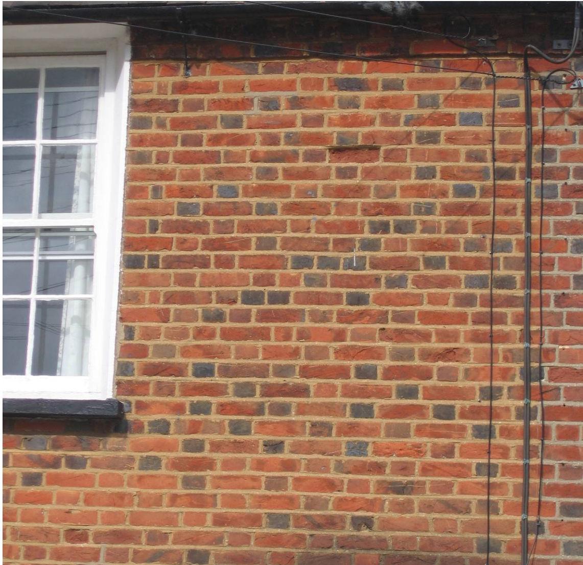
Fig. 8: Characteristic Georgian brickwork with flared headers (15-19 Cricketers Lane).
