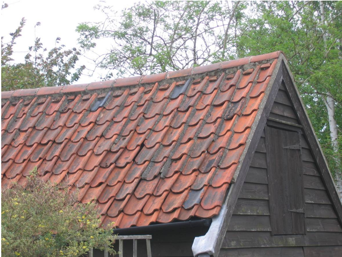
Fig. 9: Pantile roof (20 Cricketers Lane).
