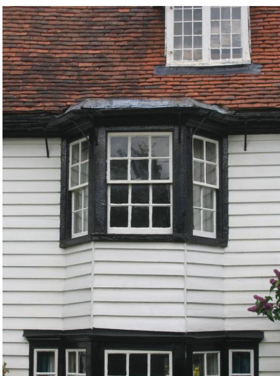
Fig. 6 (left): Feather-edged weatherboard, with a sliding sash window, beneath a roof of hand-made peg tiles (27 Cricketers Lane).
