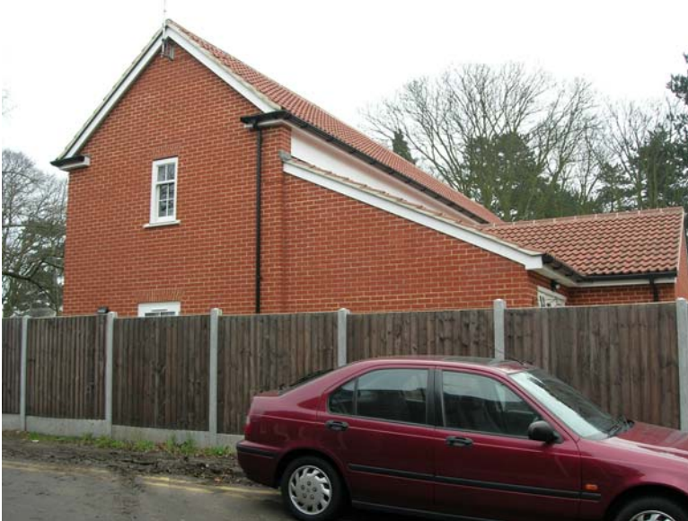
Fig. 12 Flemish bond brickwork showing brick arches and denticulated eaves
