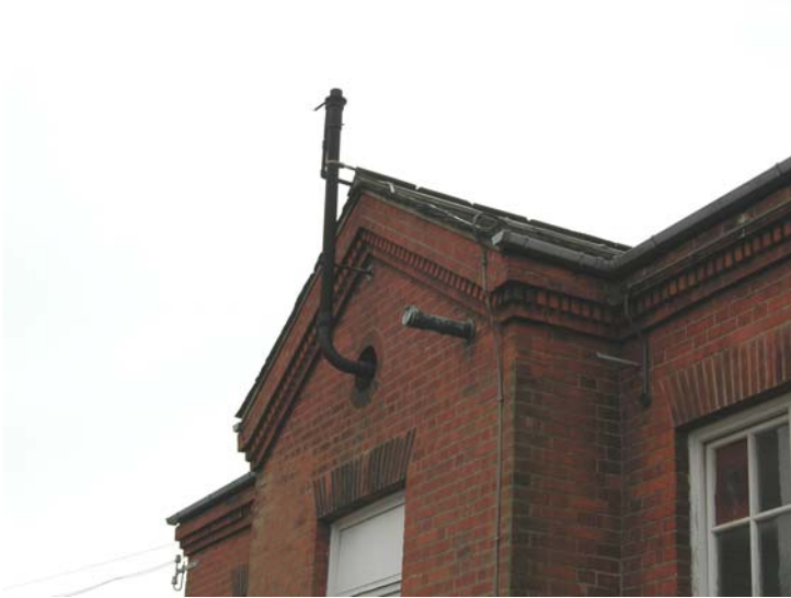
Fig. 12 Flemish bond brickwork showing brick arches and denticulated eaves
