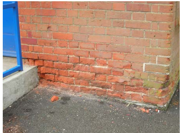
Fig. 60 loss of brickwork through change of ground level
